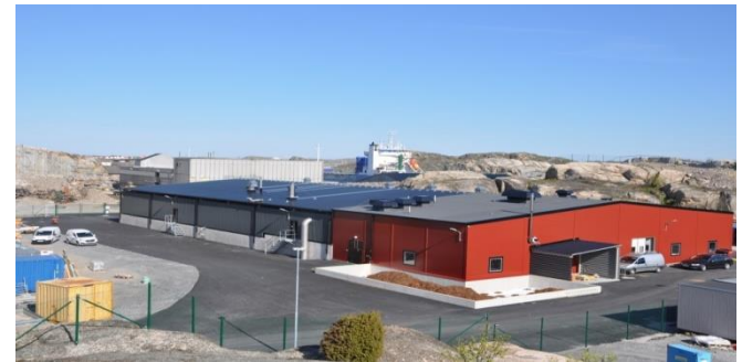
The newly built northern WWTP.
