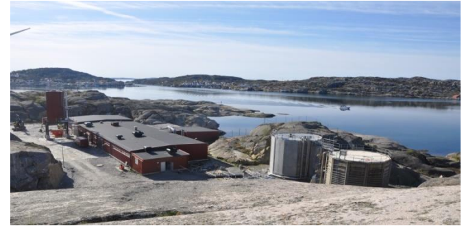
The renovated southern WWTP.
